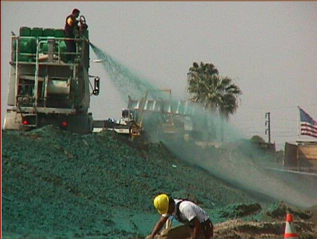
Hydraulically applied paper mulch
