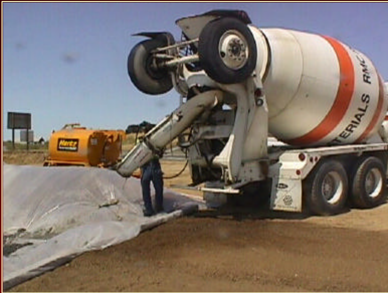
Controlled concrete washout
