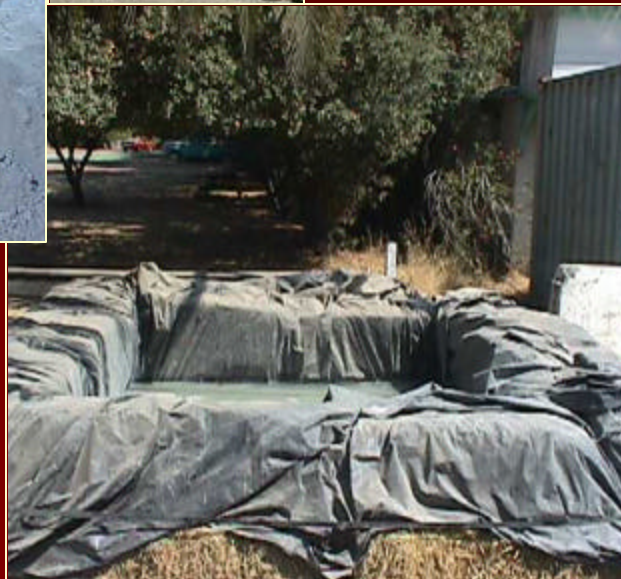
Above Grade concrete washout
