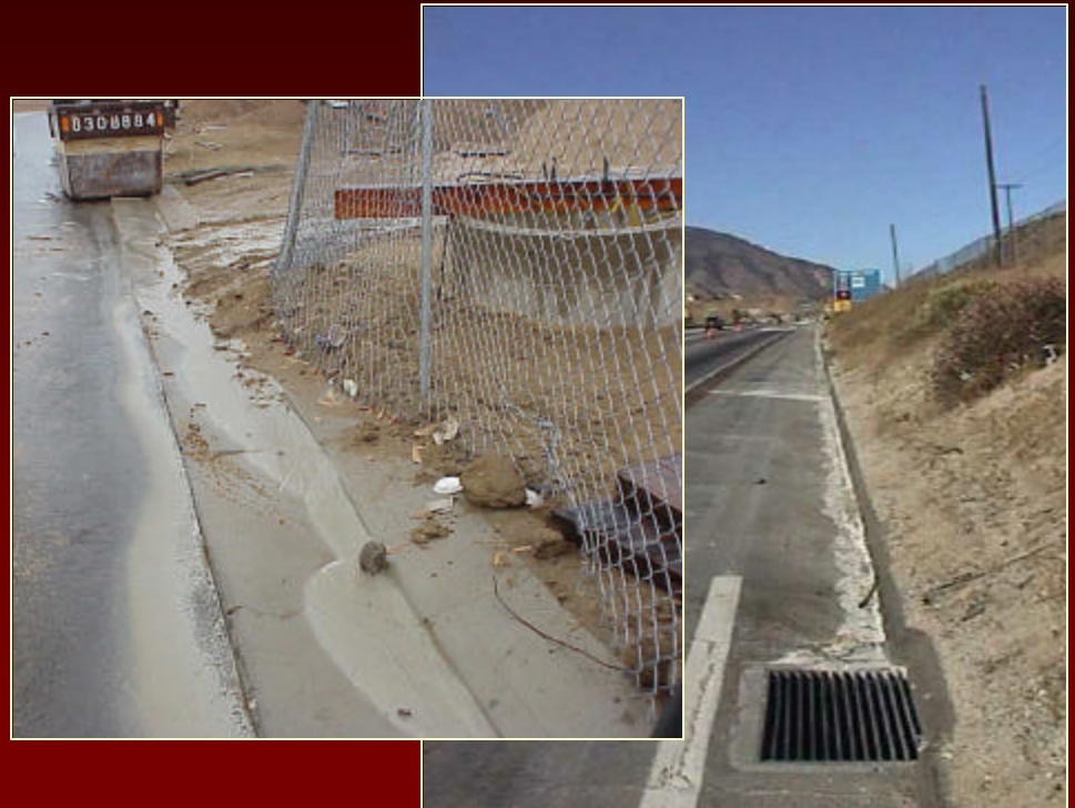
Uncontrolled concrete washouts
