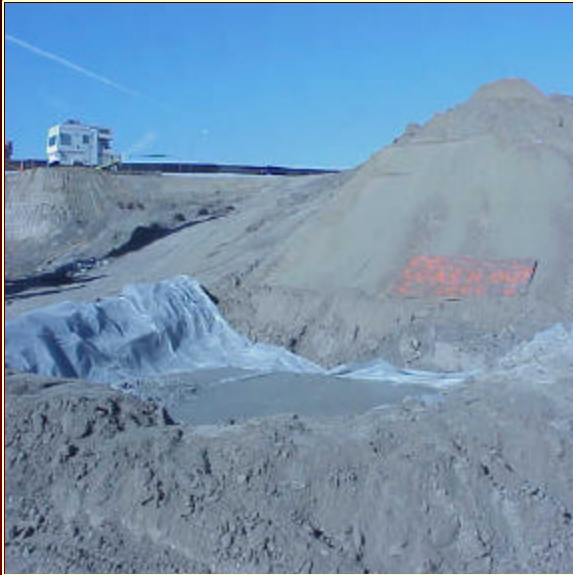
Below Grade concrete washout
