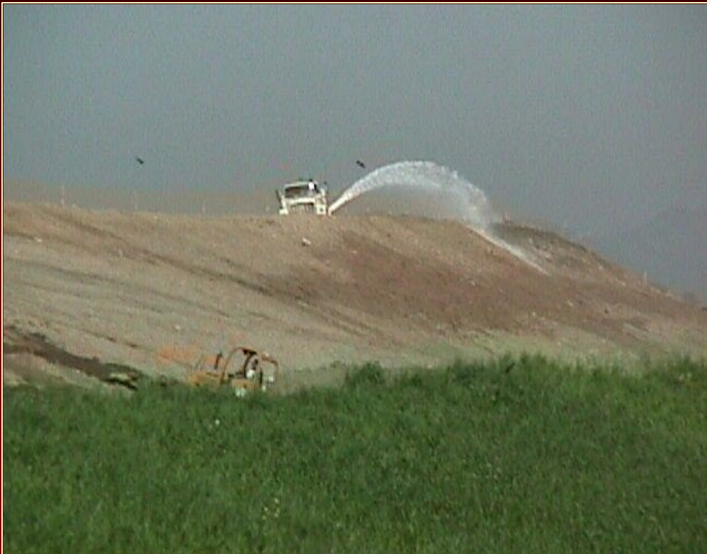
Soil binder applied via water truck
