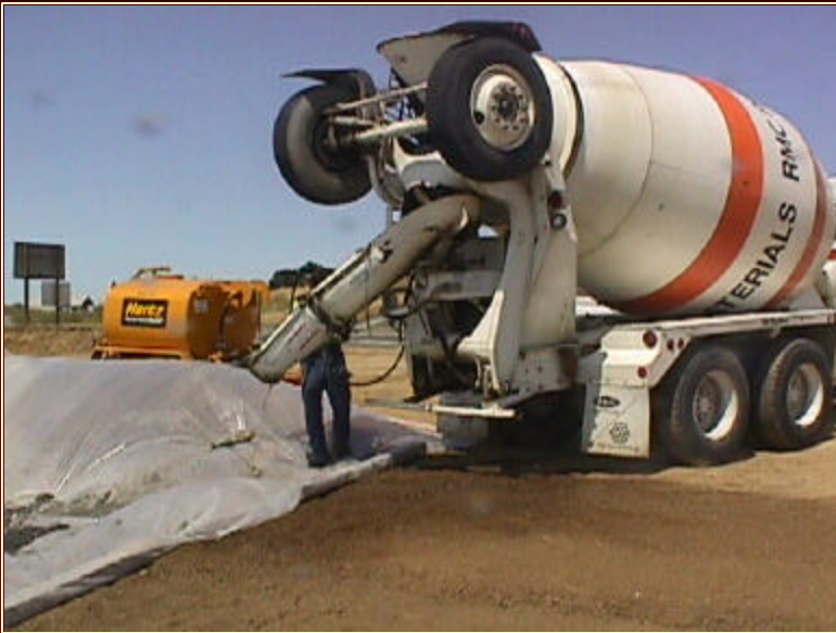
Controlled concrete washout
