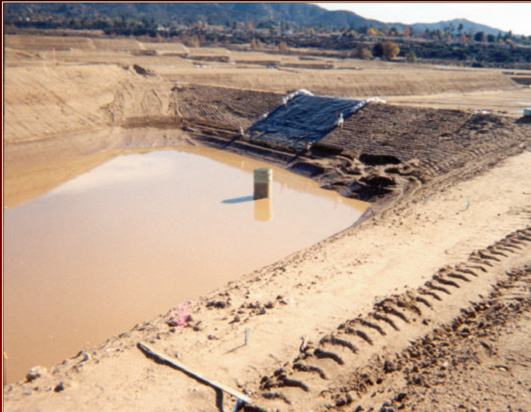
Sediment Trap without required fencing
