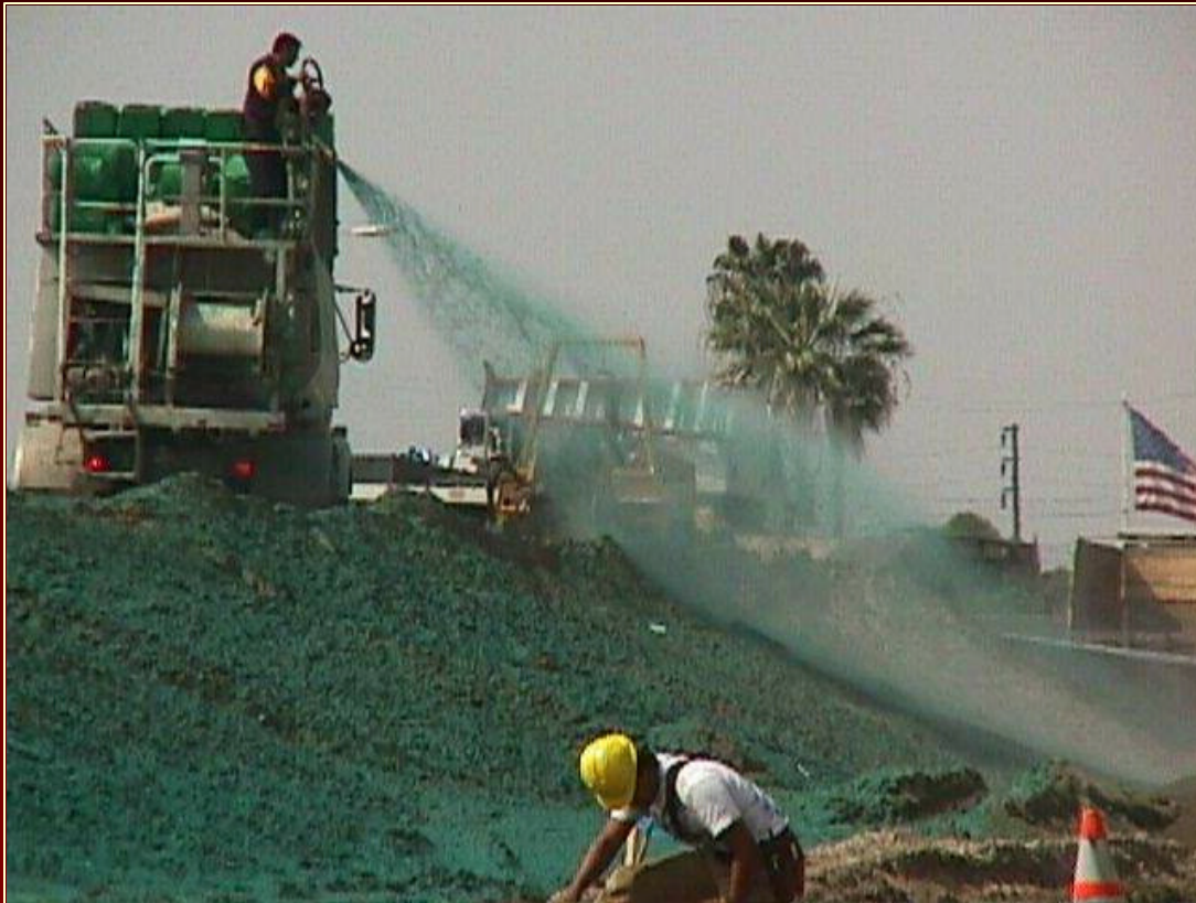
Hydraulically applied paper mulch
