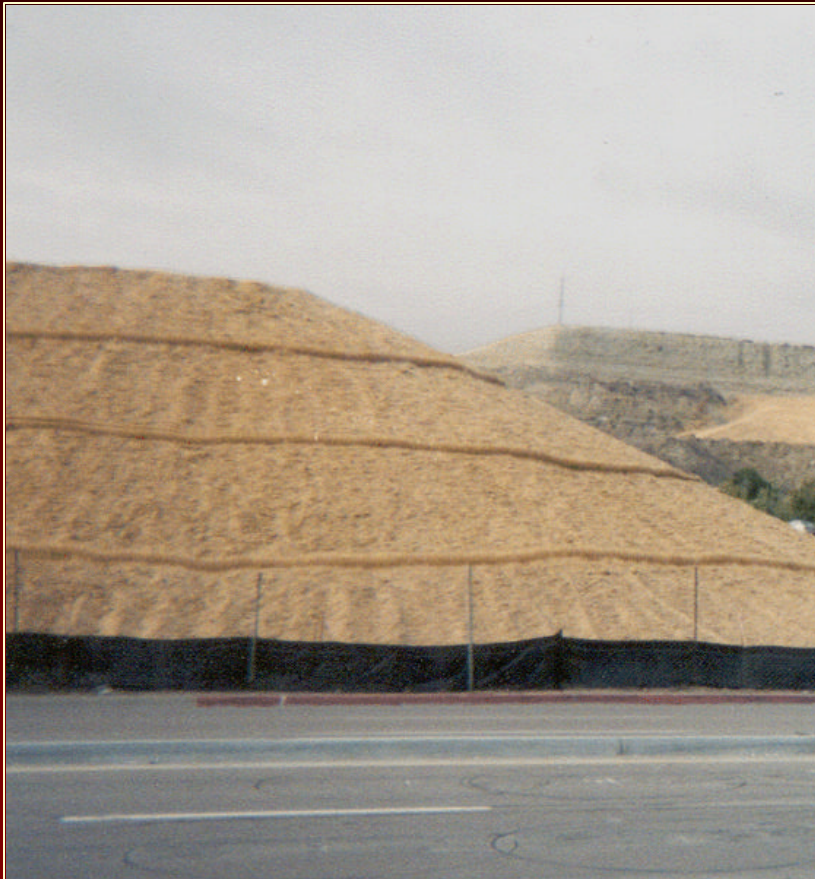
Correct installation of fiber rolls
