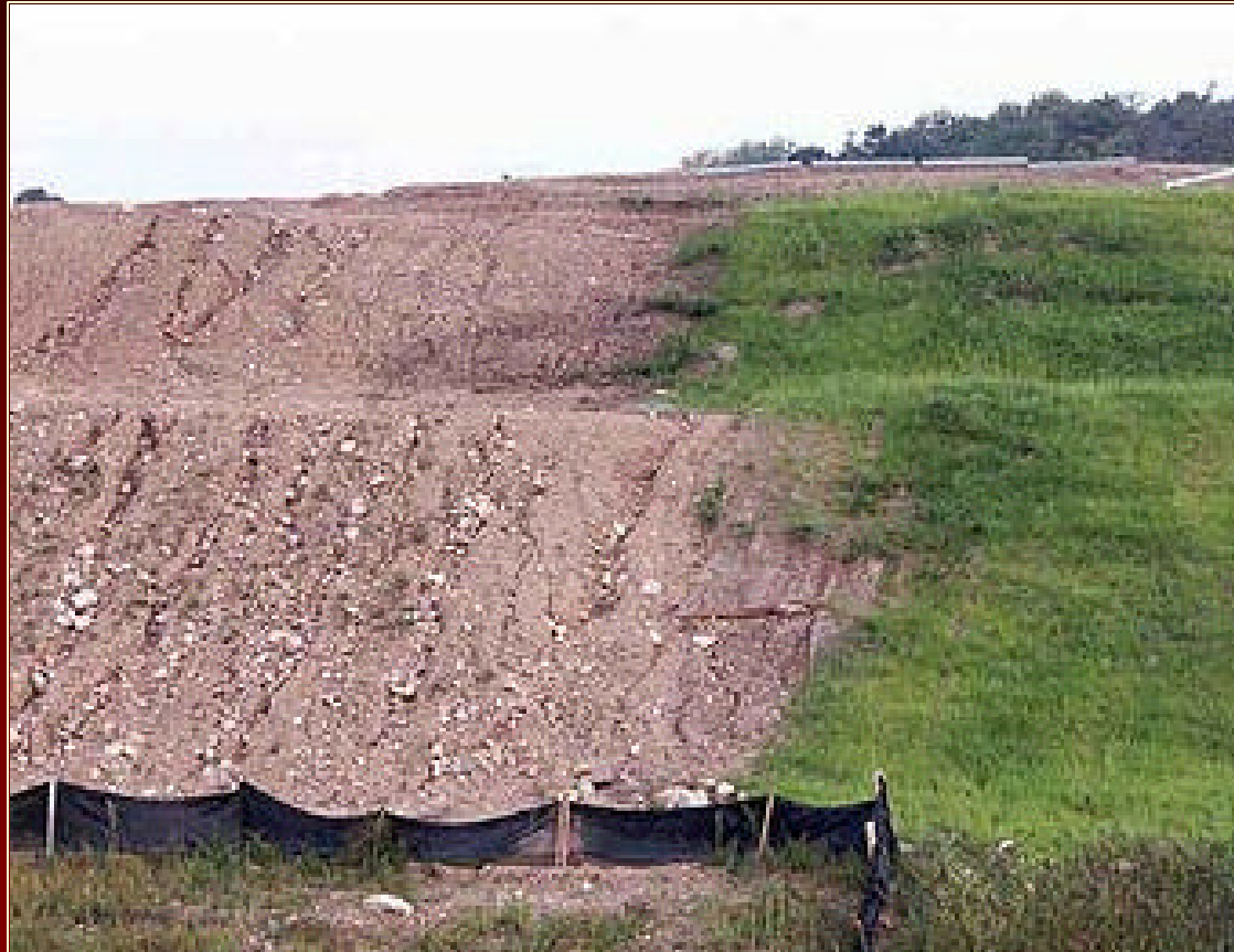
Unstabilized slope vs. Stabilized slope
