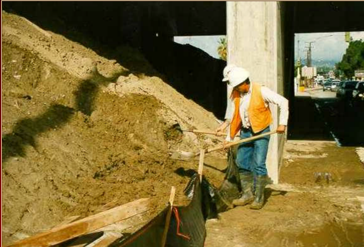
Silt fence maintenance
