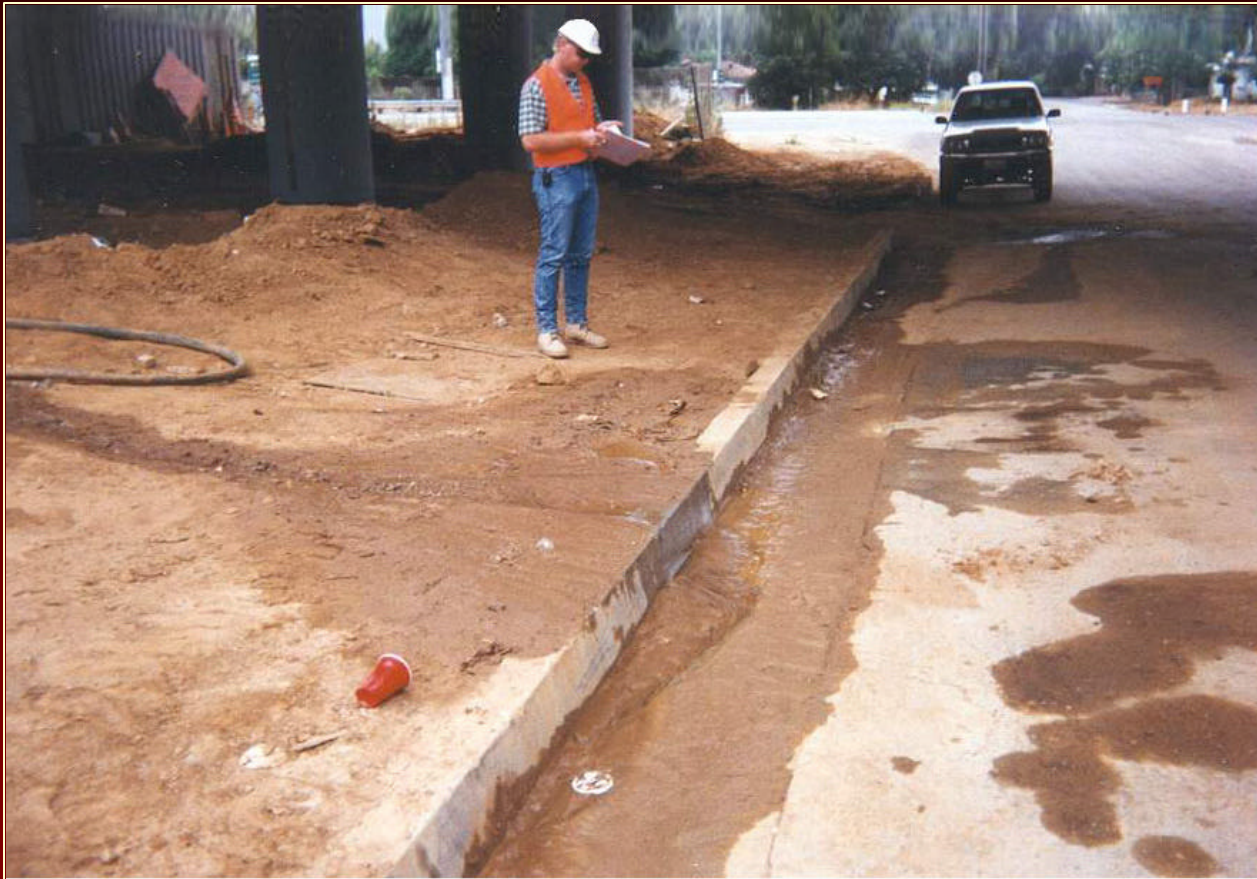
Lack of sediment control
