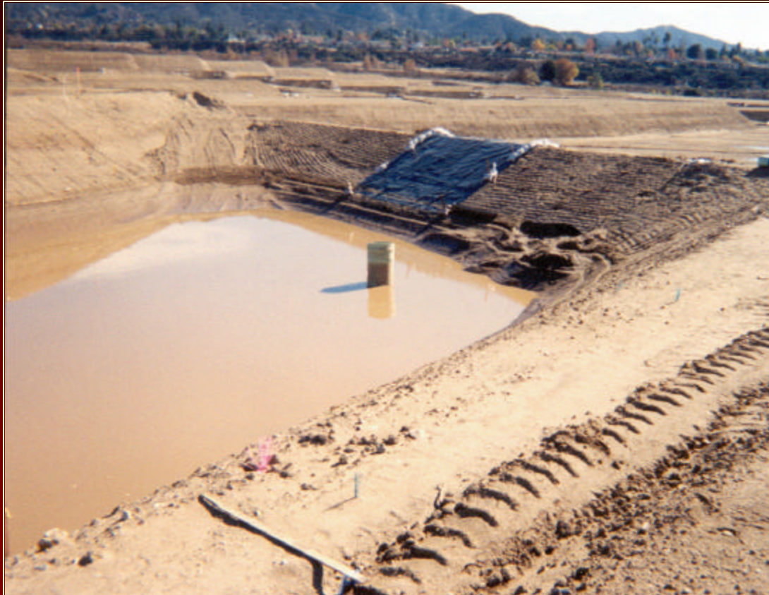
Sediment Trap without required fencing
