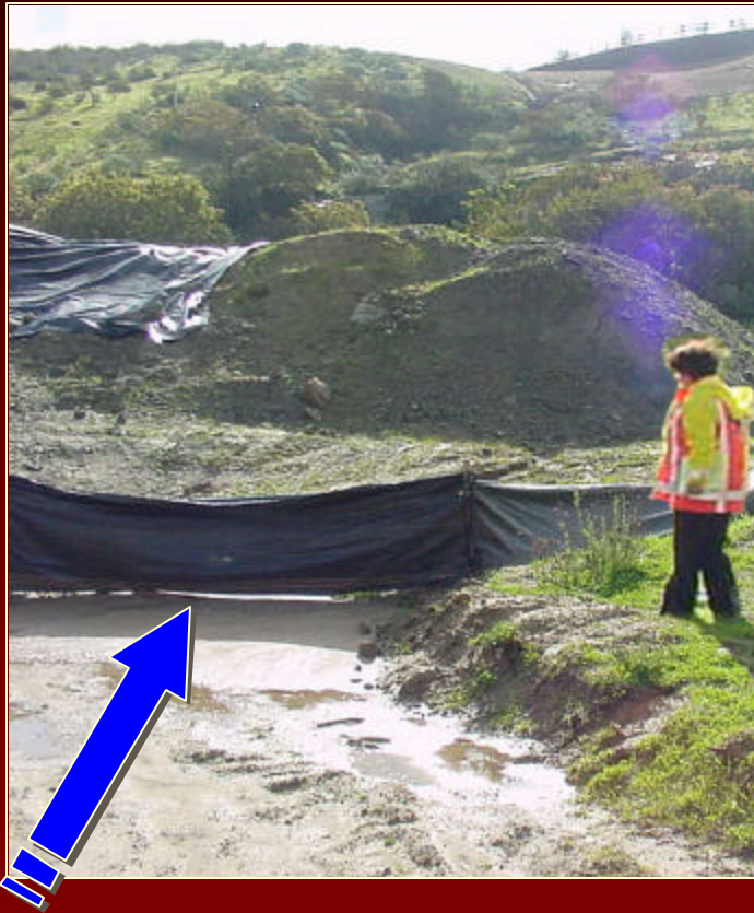
Incorrect installation of silt fence, bottom portion not properly keyed in.
