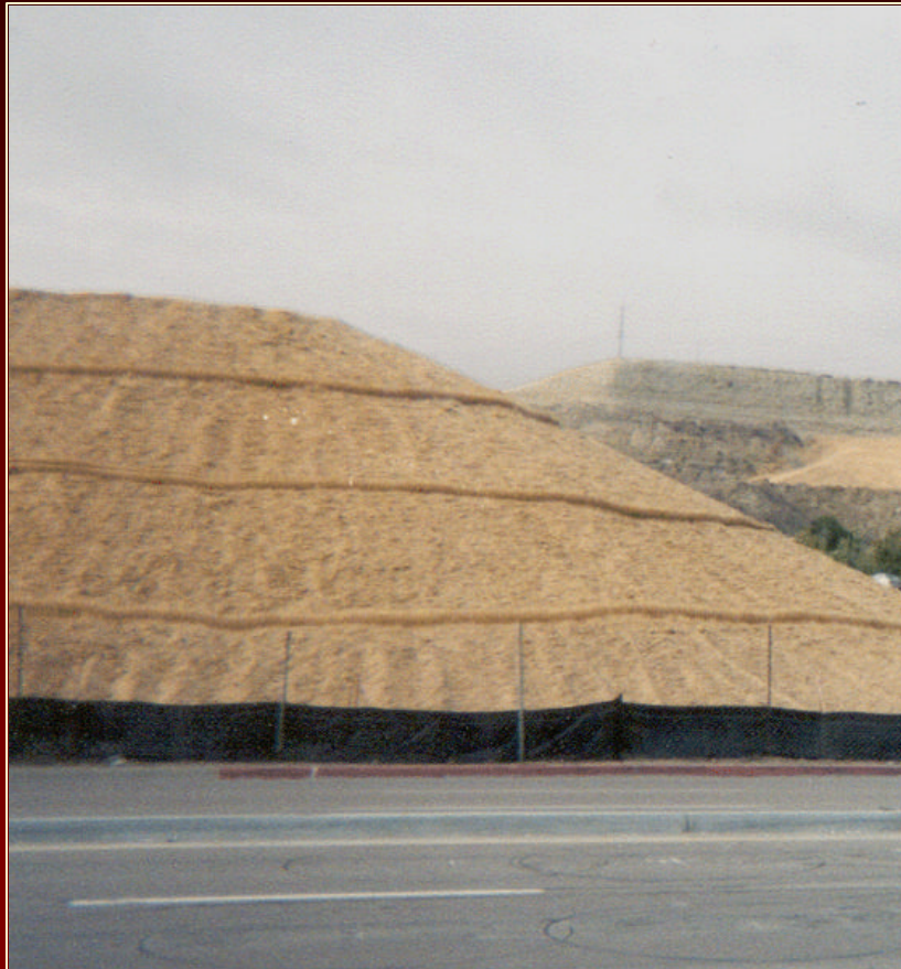
Correct installation of fiber rolls
