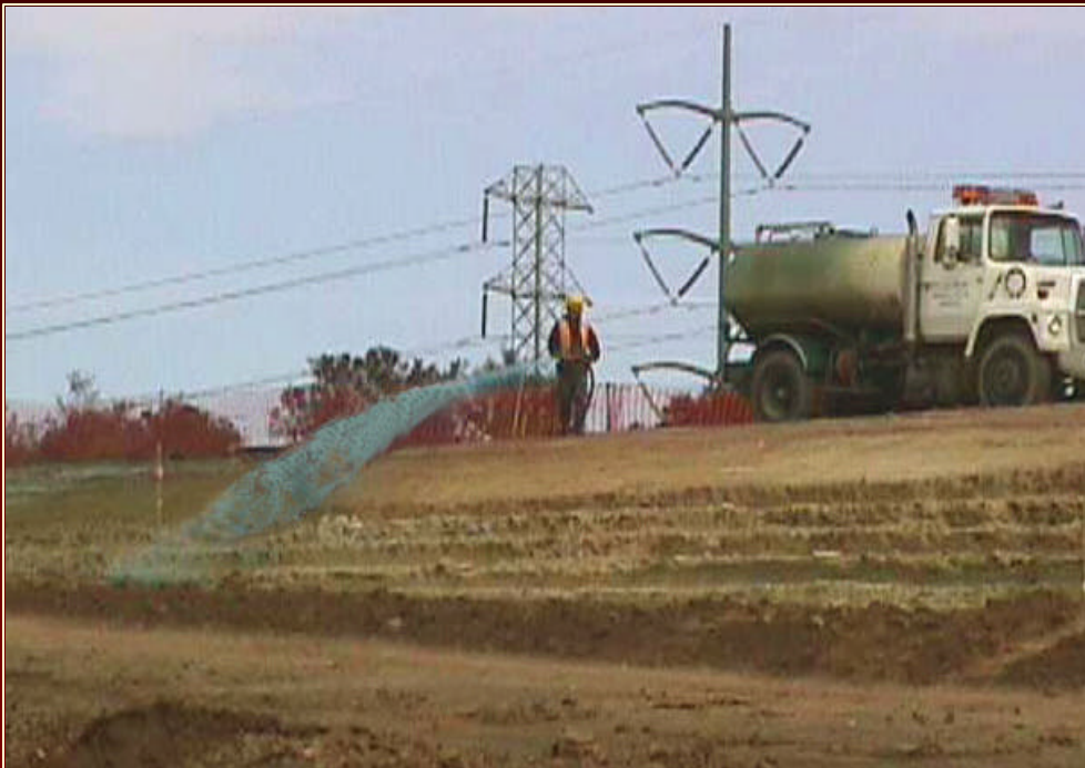
Application of Soil Binder
