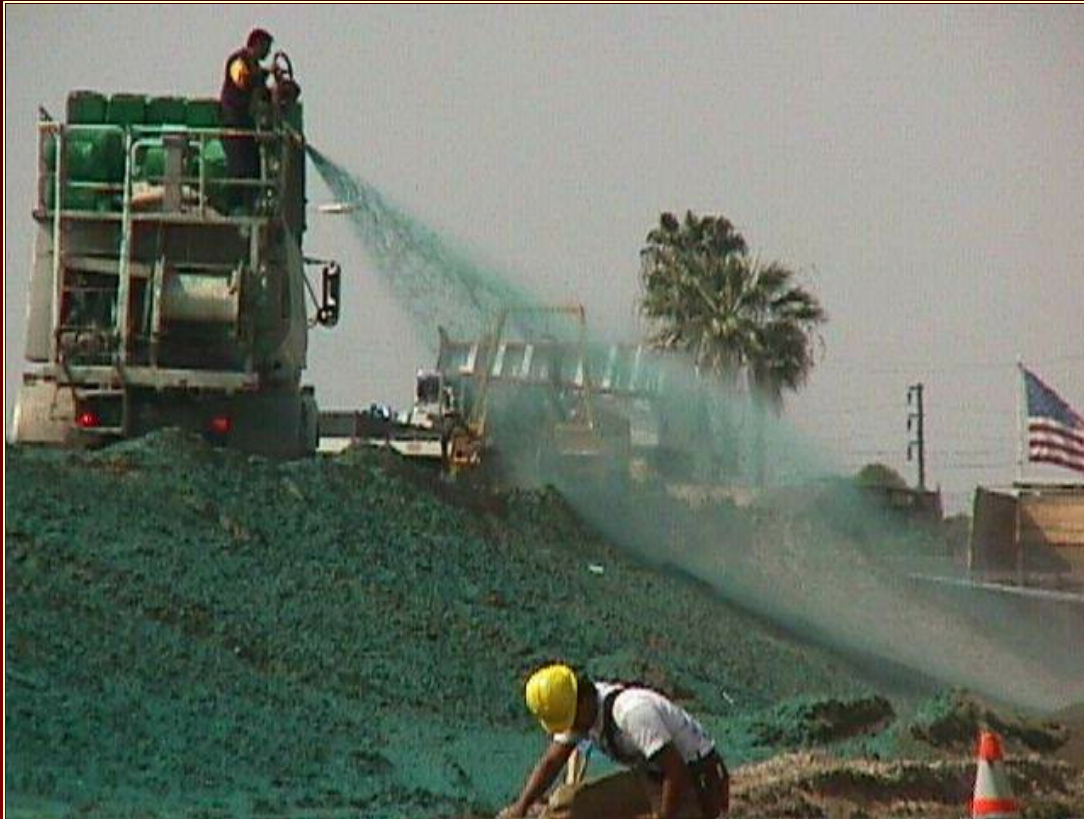
Hydraulically applied paper mulch
