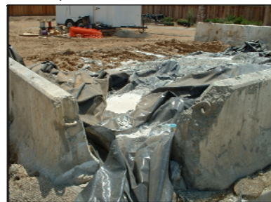
Improperly constructed washout
