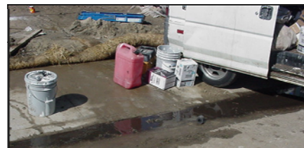
Materials should not be placed on the ground directly near conveyance systems
