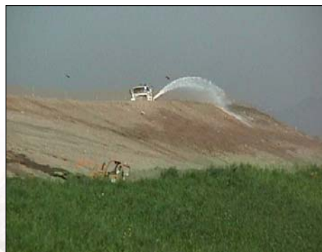
Soil binder applied via water truck
