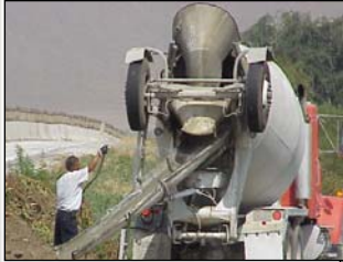
Concrete washout
