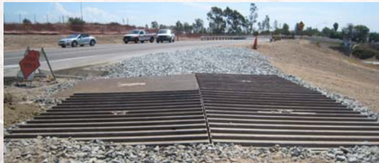
Large diameter rock used as a stabilized entrance / exit
