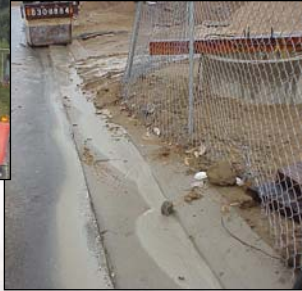
Uncontrolled concrete washouts
